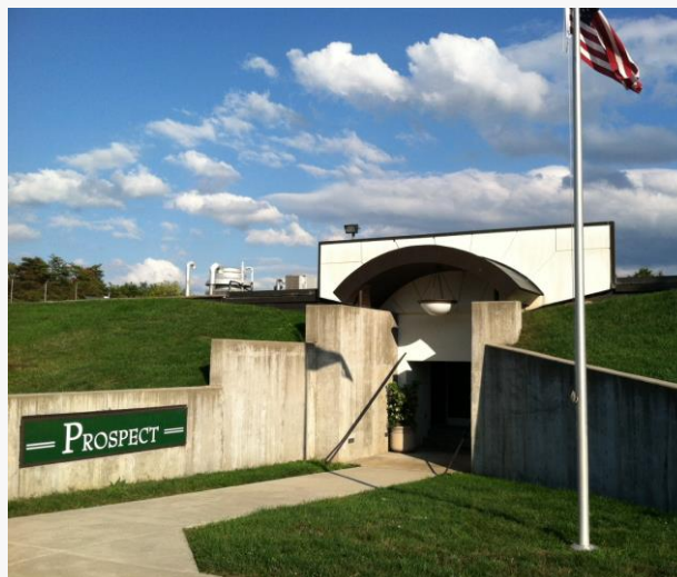
Prospect Solar's entrance to their underground building in Virginia.
