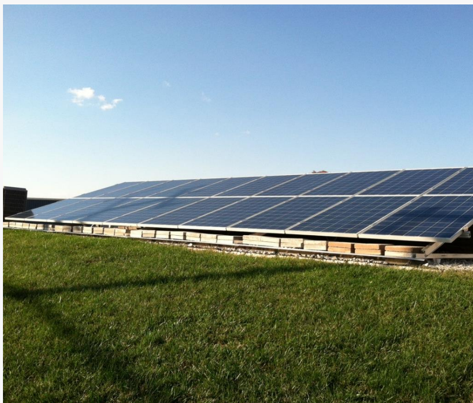
A 4.4 kw, 20-panel PV system on the roof of Prospect Solar's Sterling, VA office.
