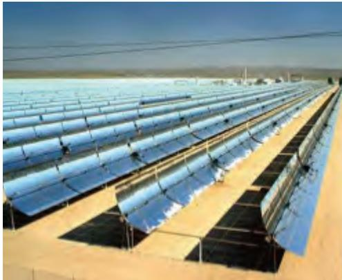
Parabolic Trough Concentrating Solar Collector at Kramer Junction, California
